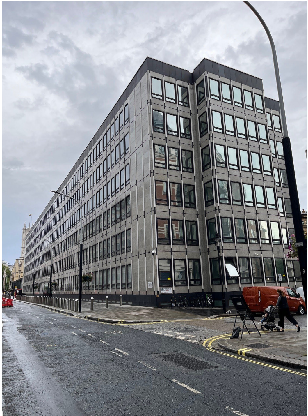
1 Victoria Street looking north-east
