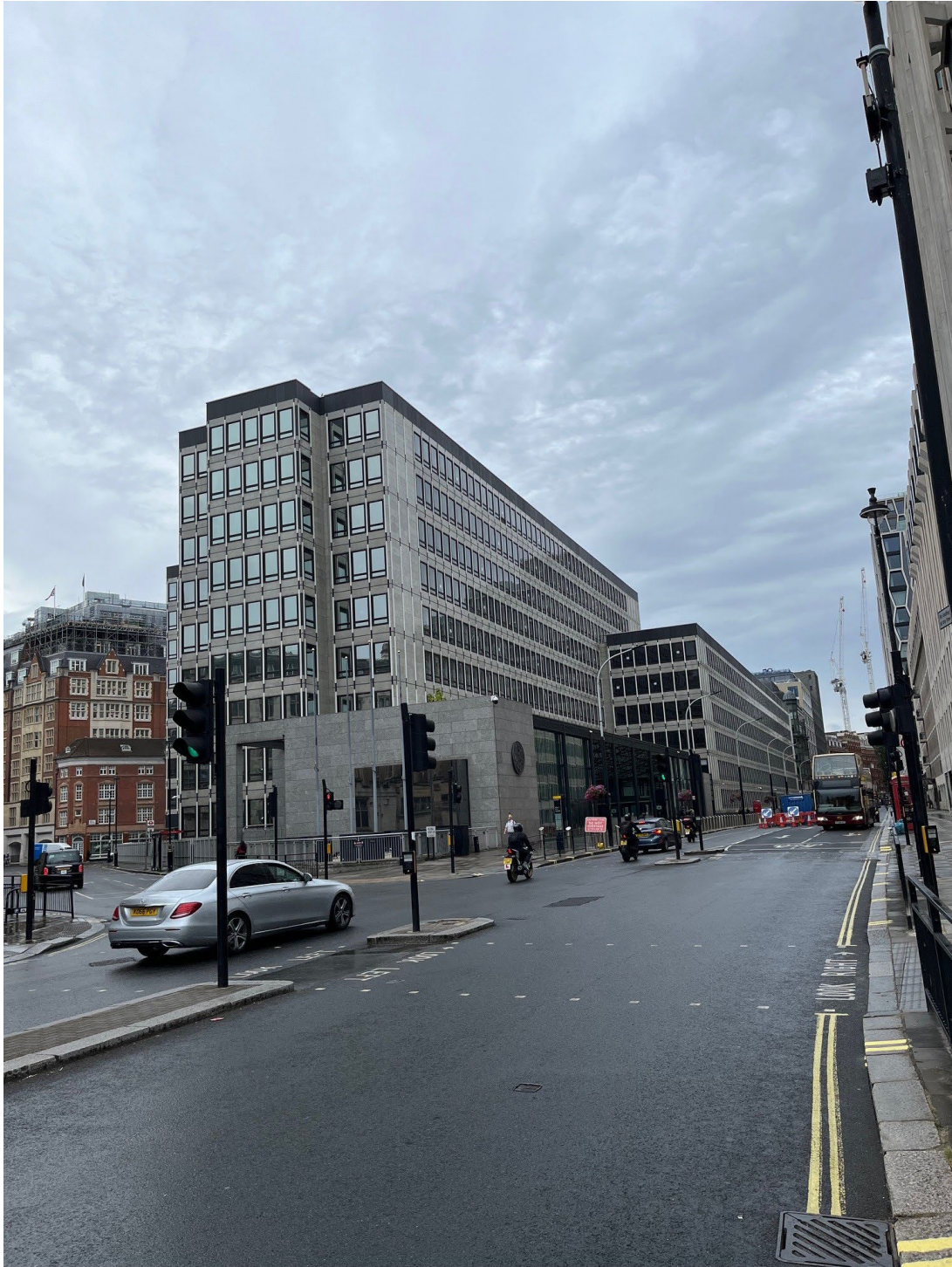
1 Victoria Street looking south-west
