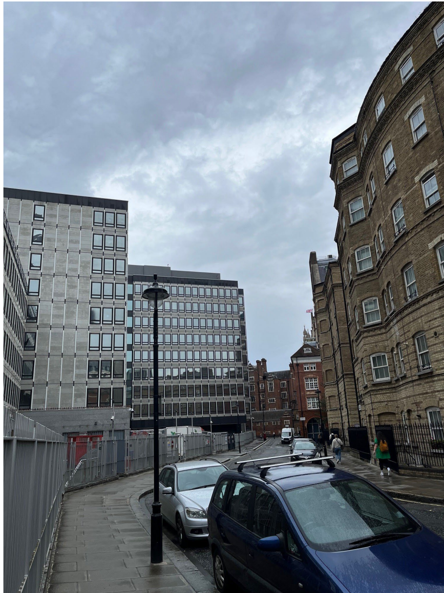
View of rear of application site along Abbey Orchard Street showing service yard.
