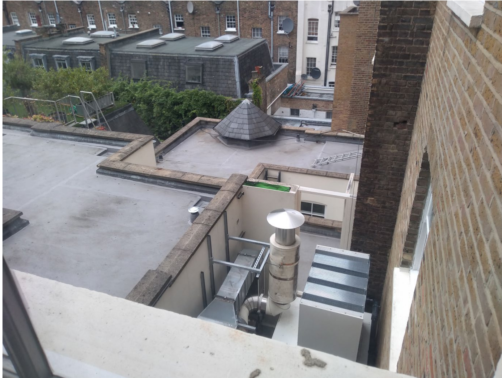
Photograph down to lightwell from window of building.
