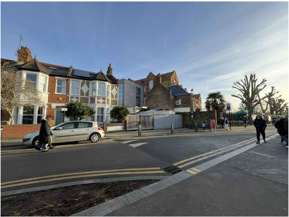
Existing Site Photographs
