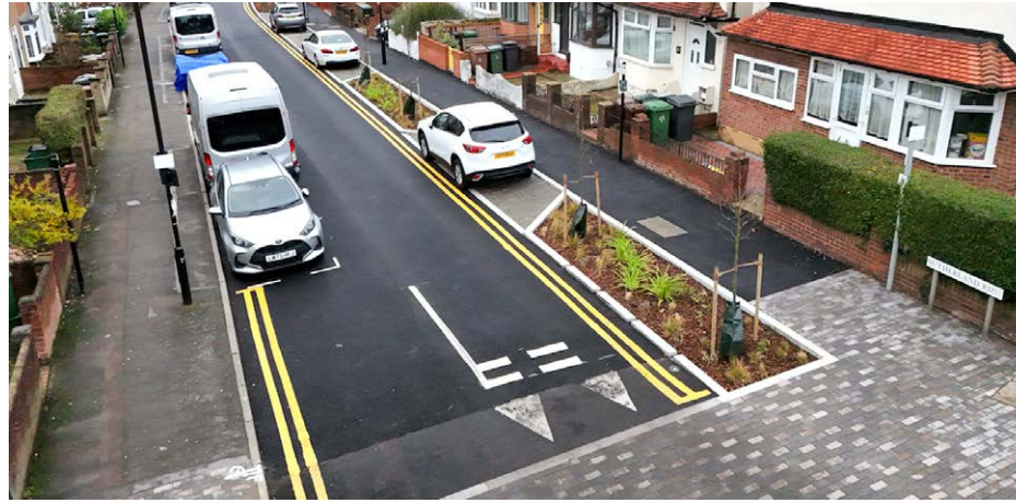
Figure 38: Sutherland Road planting and road upgrades completed
