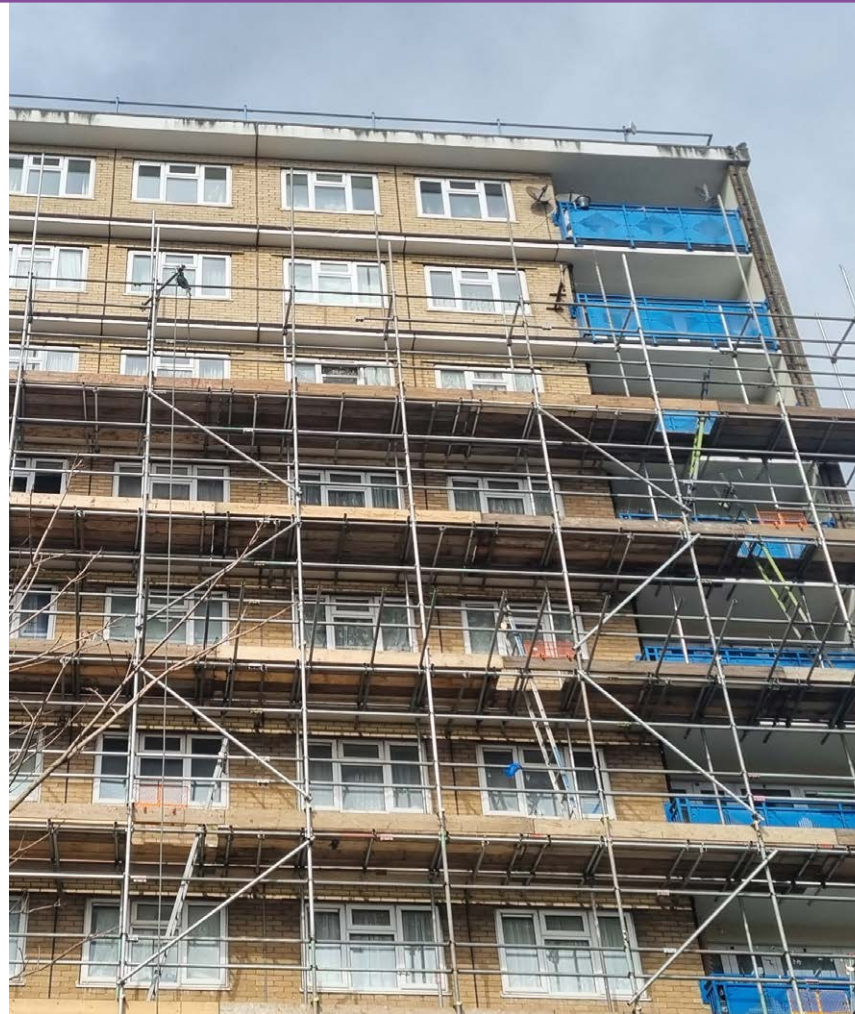
Figure 28: Building safety works underway
