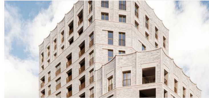
Figure 12: New affordable homes at Precision House, Wood Street
