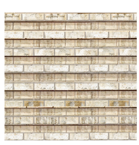
Feature Brickwork: Projecting brick stripes
