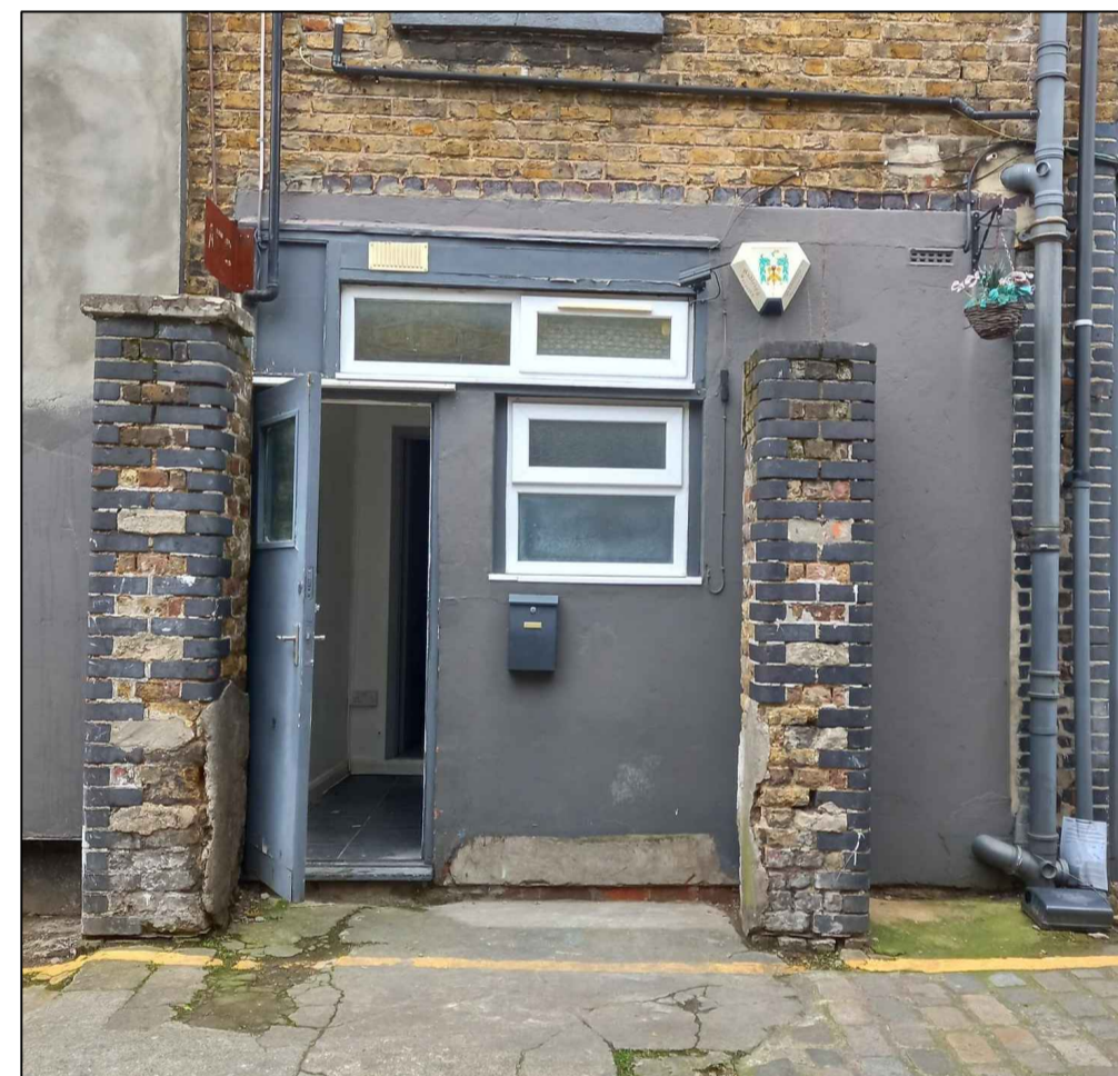
UNIT 37A SHOP FRONT
