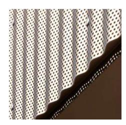
Example of perforated metal screen with wave profile Welltec W-8/25 by Cadish MDA or similar. Panel and frame colour: light green to match window frame.
