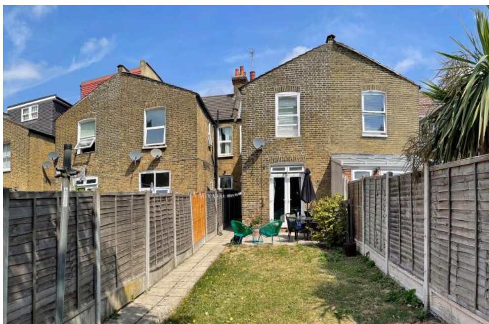
Photo showing rear of proposal property, No. 5 with the rear extension and No.9
