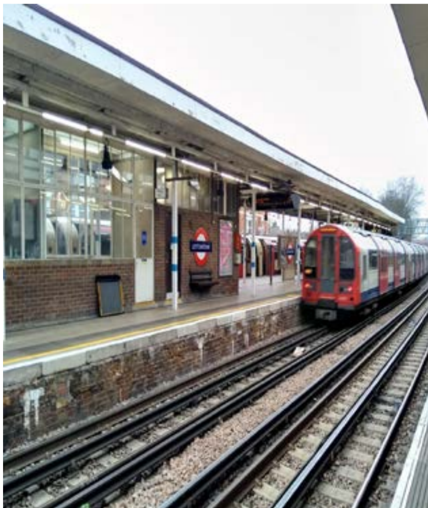
Leytonstone Underground Station
