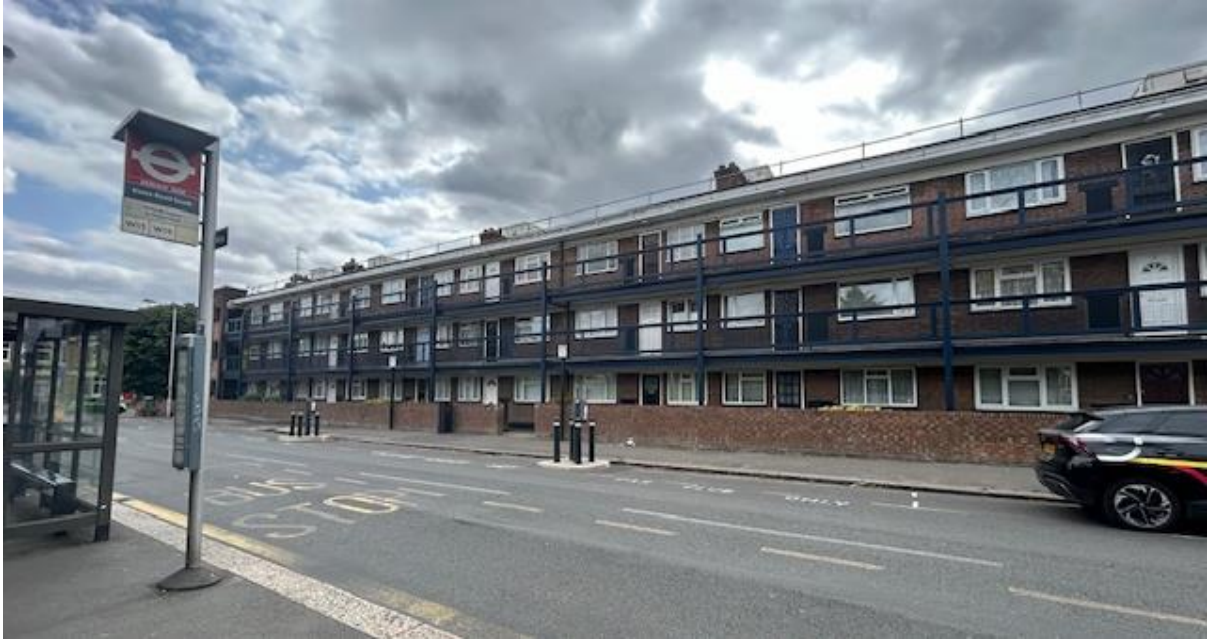
The existing building as viewed from the north east side of Essex Road.
