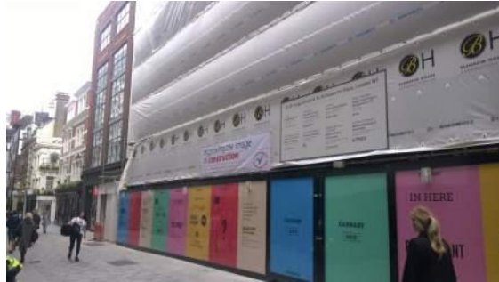
Figure 13: Example of Secure hoarding to perimeter of the site.
