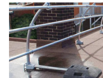
Precedent of the maintenance guardrail
