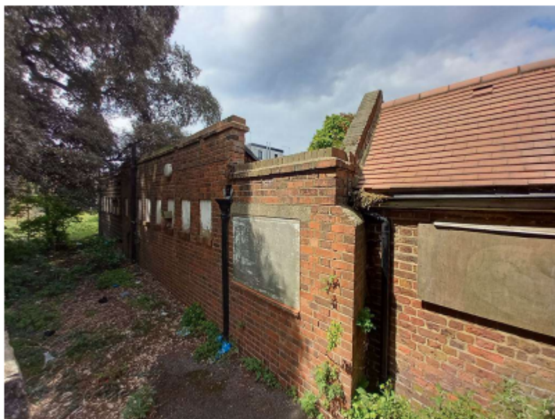
Ground level view of the flat roof section to be removed.
