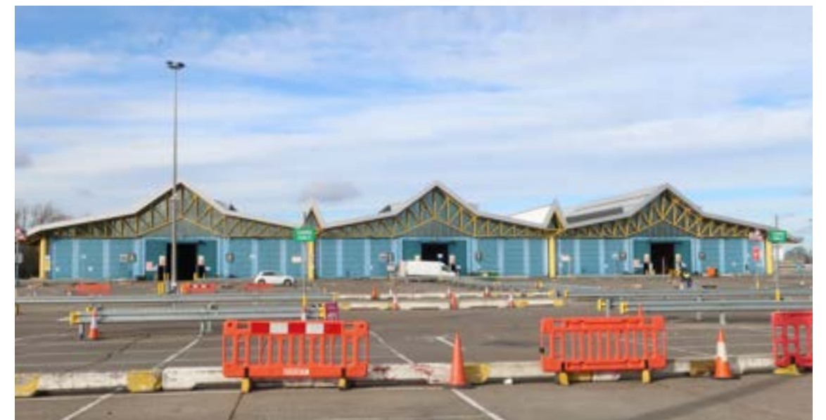
Image 61. The existing market hall at New Spitalfields Market - once the market vacates, the framed structure could accommodate meanwhile uses.
