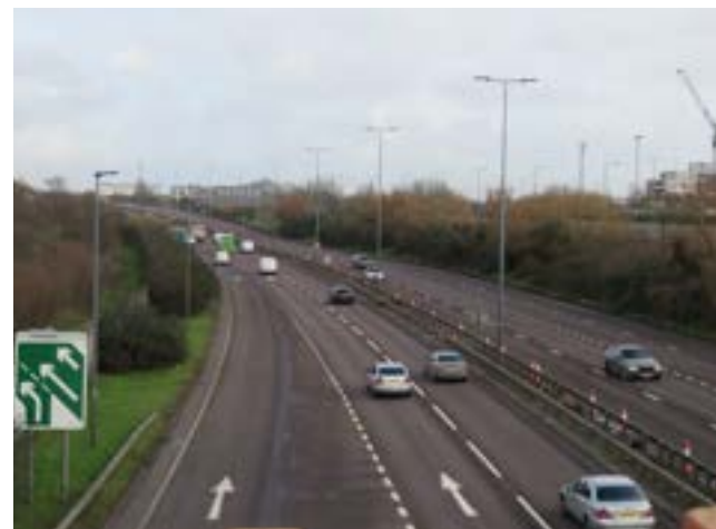
Image 15: Severance caused by A12
