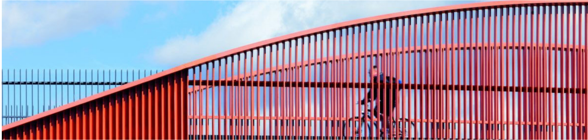
Image 18: The existing cycle and walking bridge over Eastway into the Queen Elizabeth Olympic Park (Allies and Morrison) A great example of new cycling and walking infrastructure that overcomes severance, joins up with a wider network and is beautifully designed.
