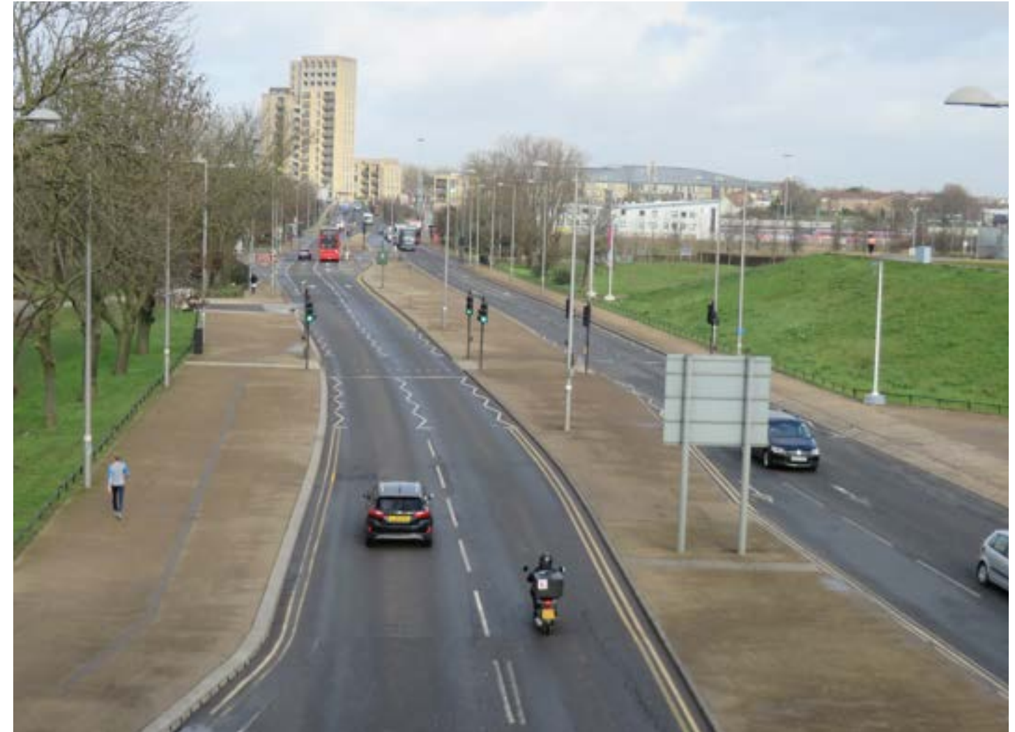
Image 14: Severance caused by A06 Eastway. Potential improvements along staggered crossings and for designated cycle lanes along Eastway by reconfiguring central reservation
