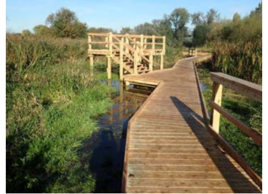
Image 63. Boardwalk along the de-culverted River Wandle, Wandle Park, Croydon
