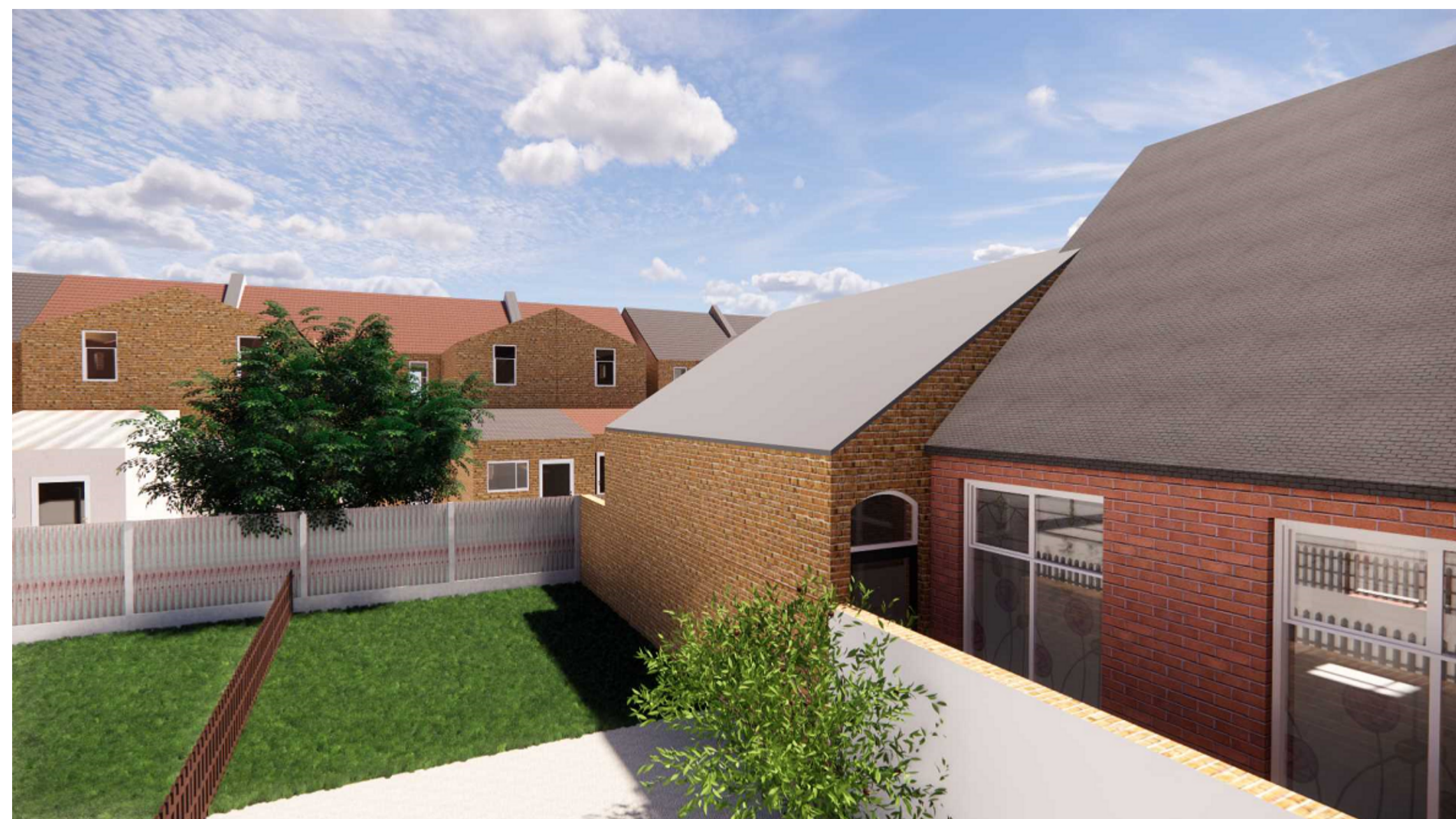
View of the existing church roof from 12A Hainault Road - First Floor
