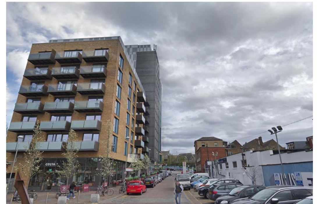
View To Site On Station Approach
