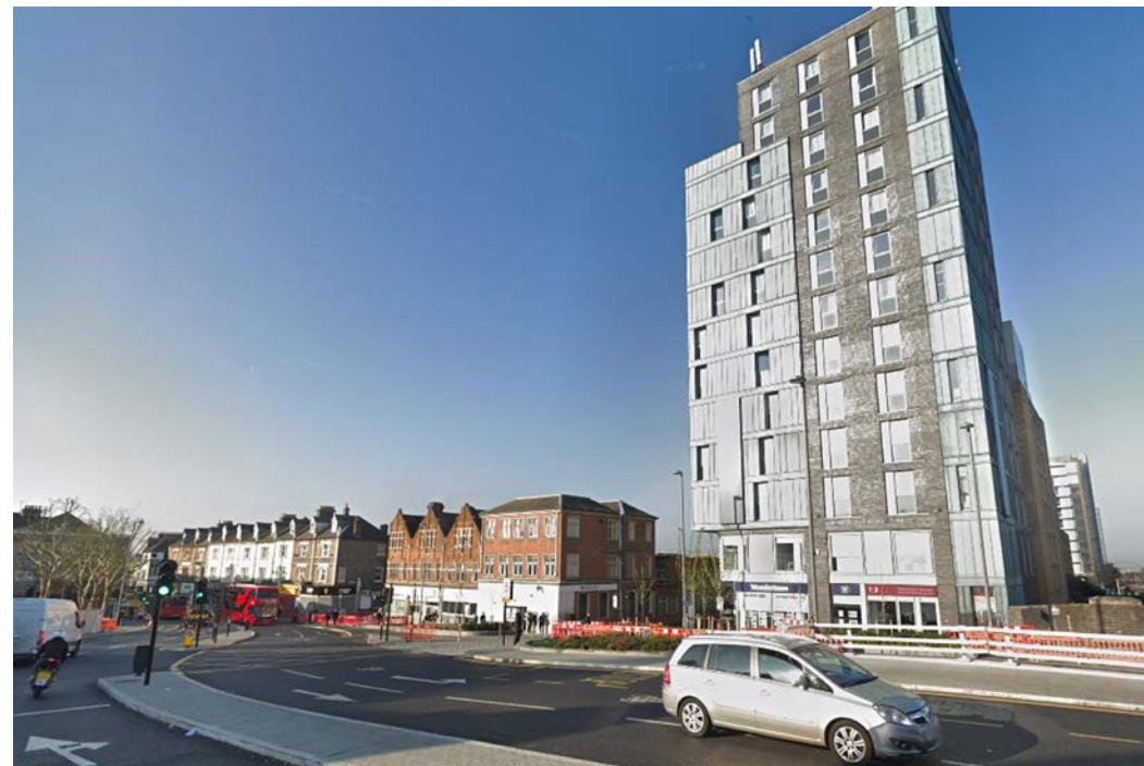
View Looking South To Site From Hoe Street
