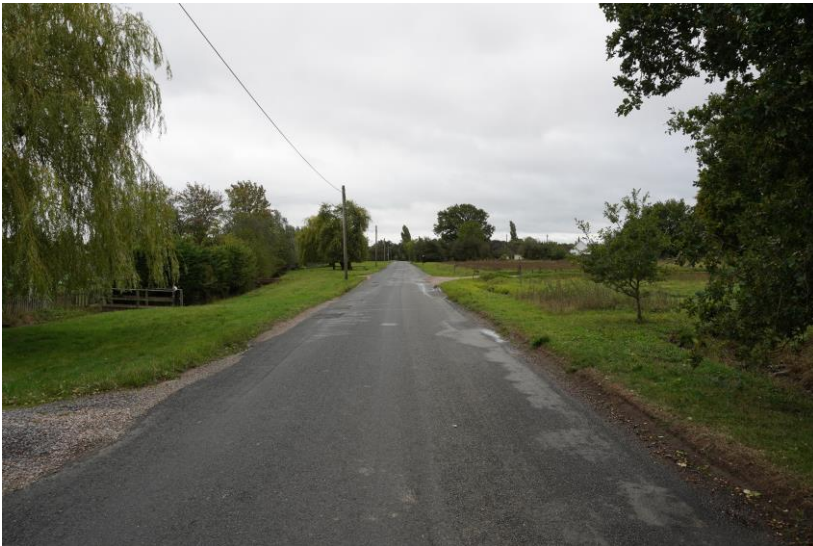
Figure 18 View 3 looking southeast from the centre of the Conservation Area
