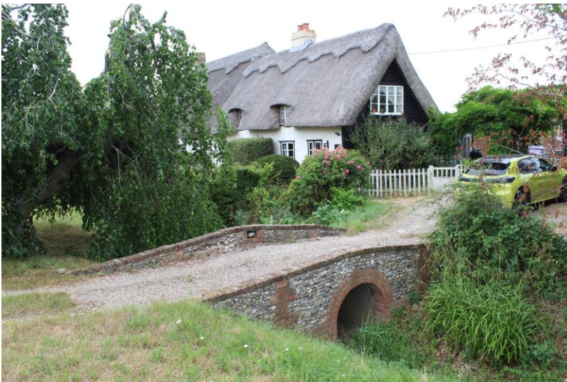
Figure 13 Flint and brick bridge over the River Ter leading to Byways & Sunnyside
