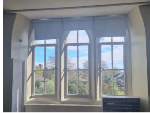
Photo 11: Example of a metal framed single glazed window, no secondary glazing
