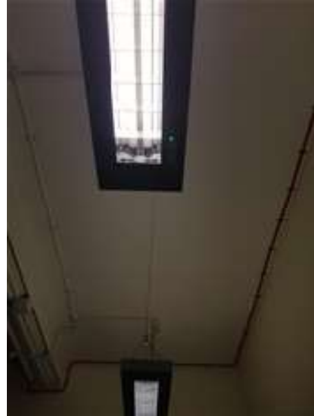
Photo 23: Surface T8 luminaire and integral emergency
