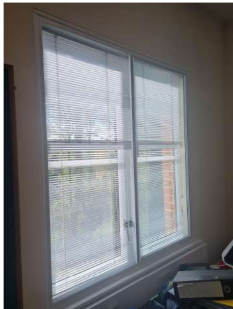
Photo 15: Example with secondary glazing with blind (Office 27)
