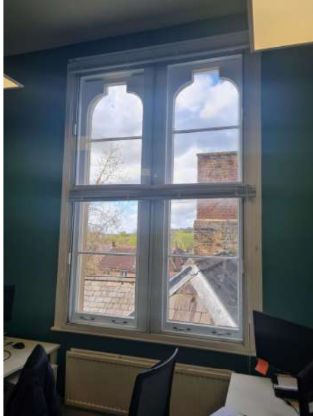
Photo 10: Example of a single glazed timber window with secondary glazing
