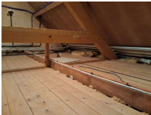
Photo 6: Roof void above Office RM 24.1 with no insulation
