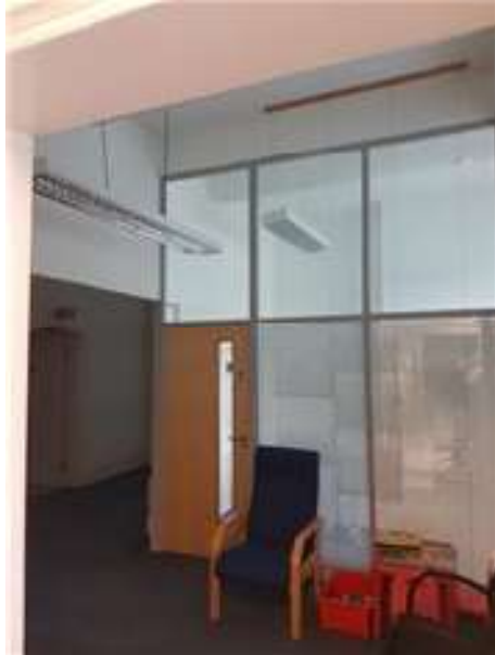
Photo 22: T8 suspended modular luminaire
