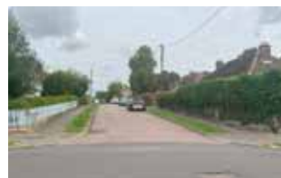
Figure 5.15. Example of narrow, sloping footway alongside busy road (top), example of side road junction with no tactile paving (bottom)
