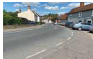
Figure 6.16. Example of 'disappearing' footway on one side of the road with no crossing point for pedestrians to cross the road
