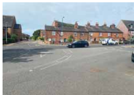
Figure 6.11. Example of confusing junction layout with multiple entry lanes
