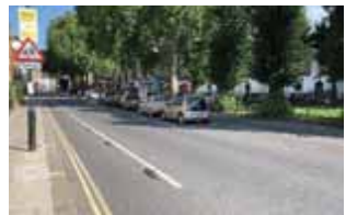
Figure 5.16. Example of light segregation where highway width is limited (Royal College St, Camden)
