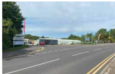
Figure 6.10. Example of wide side road junction without tactile paving
