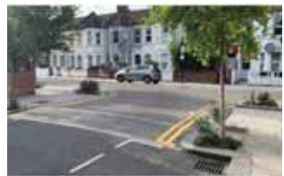
Figure 5.18. Raised table crossing of side-road (Devon Gardens, Harringay)
