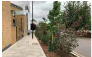
Figure 6.19. Clear footway incorporating SuDS (Crossway, Hackney)
