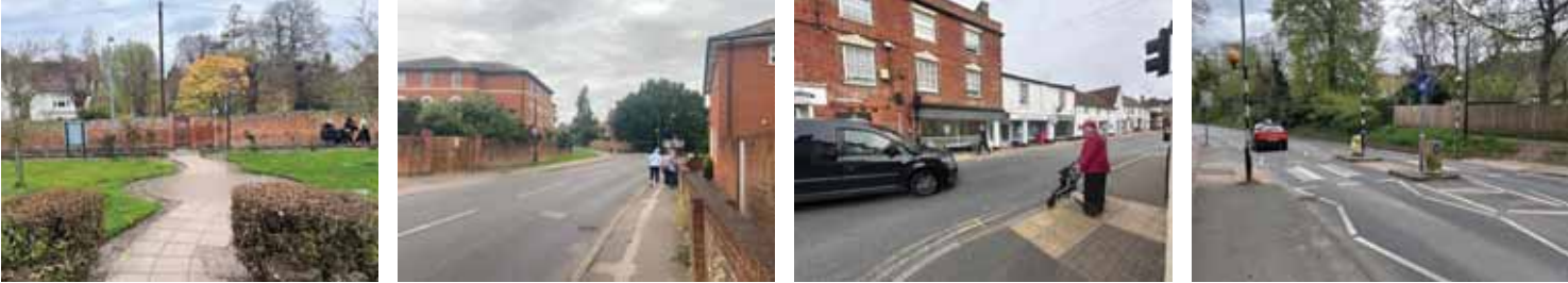
Figure 5.2 Footpaths and cut-throughs create a porous pedestrian network in the town (left); footway widths commonly are less than 2m; pedestrian waiting to cross a busy road at a controlled crossing; example of zebra crossing to address severance (right)
