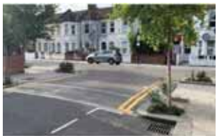
Figure 5.18. Raised table crossing of side-road (Devon Gardens, Harringay)
