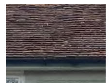
Peg tiled roof
