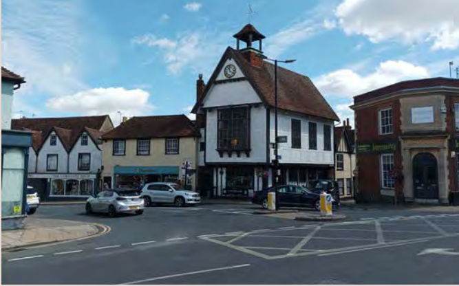
▲ Peg tiled roof, casement windows, and historic detailing on Market Street.
