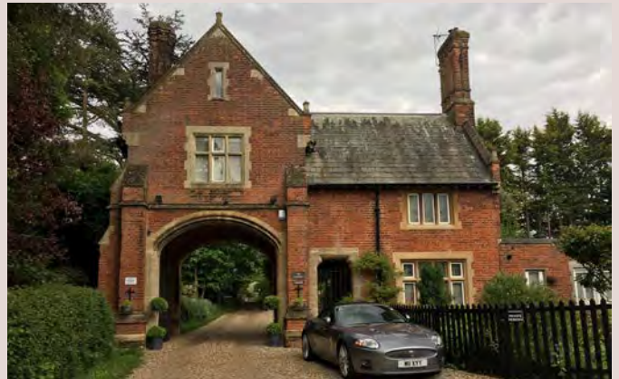
▲ Red brick gatehouse building typology with carriage-arch.
