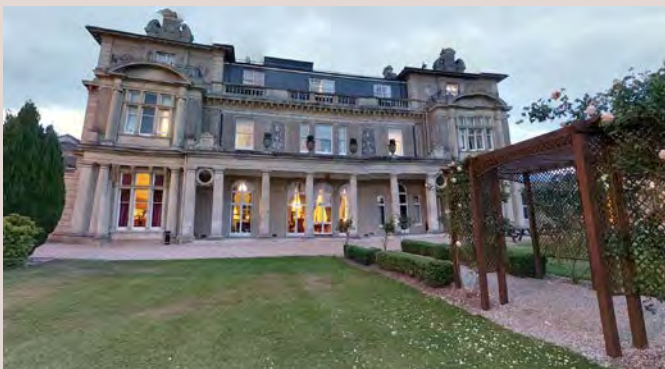
▲ Three storeyed manor house at Down Hall, Hatfield Heath.
