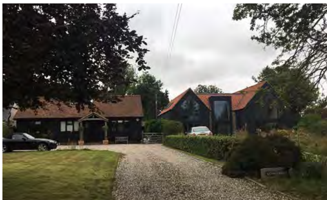
▲ Use of black timber referencing surrounding farm buildings in Duddenhoe End.
