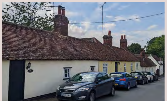
▲ Single storey timber framed terrace houses decline in line with topography creating variation and interest to the street scene in Newport.
