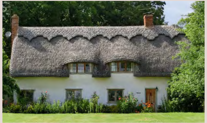
▲ Dormer windows on the 17th Century thatched cottage in Takeley.
