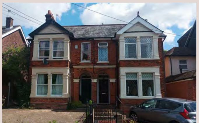
▲ Order and symmetry with Edwardian paired semi-detached houses with red brick and arched doorways on Station Road.
