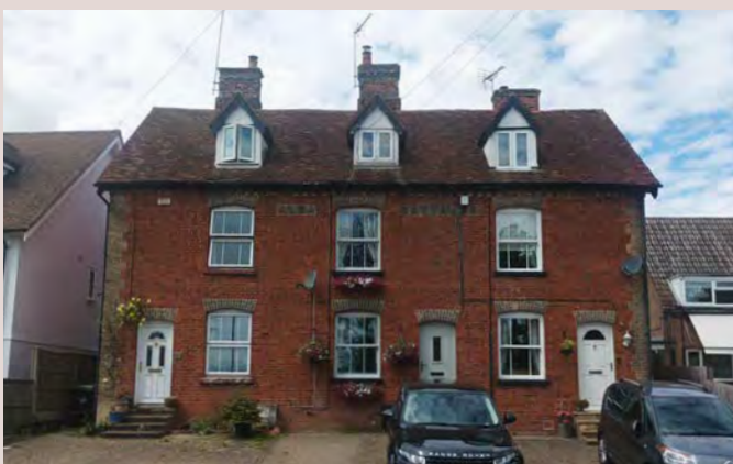
▲ Dormer windows and central stack chimneys create strong character for red brick terraces.
