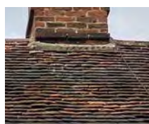
Peg tiled roof
