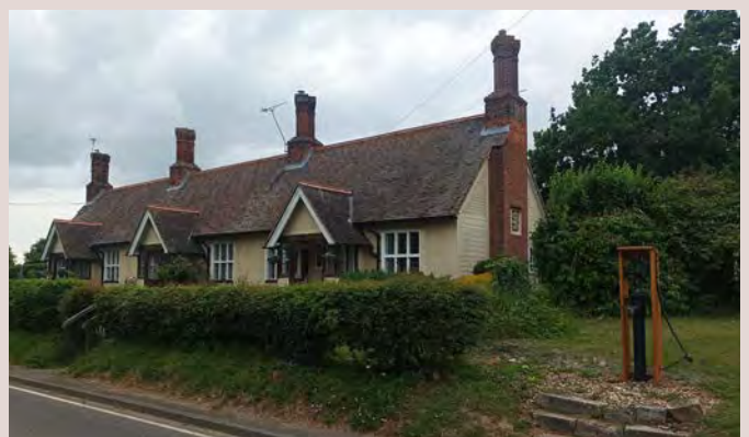
▲ Almshouses in Radwinter - Three gabled porches project on the front. Roofs tiled, with 4 chimney stacks each and casement windows.
