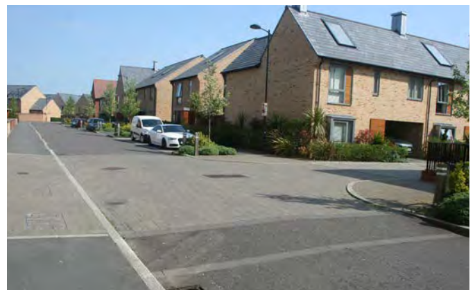
▲ Overlooked on-street parking that uses landscaping to soften the visual impact of cars and to control anti-social parking.
