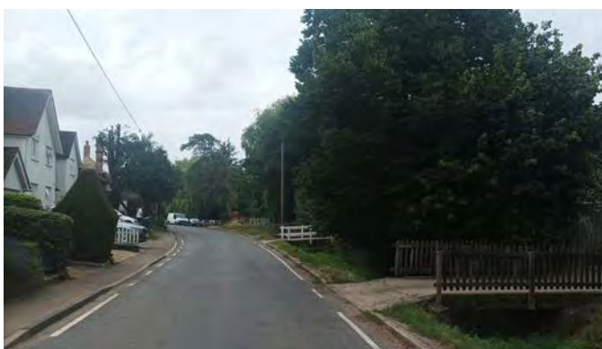
▲ Access to individual driveways successfully integrates with the swale that runs alongside the main street in Arkesden.
