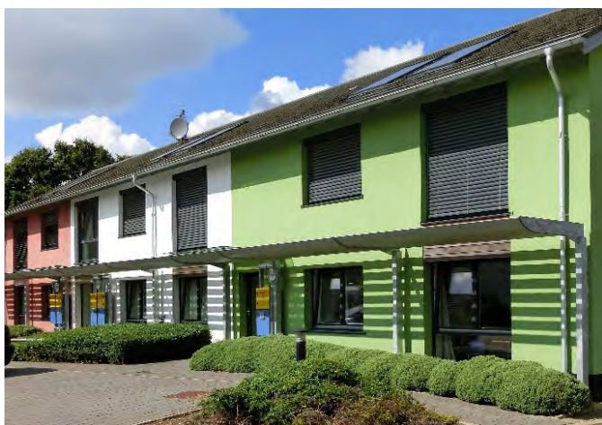
▲ Passivhaus development in Wimbish development where the properties are reserved for applicants with a strong local connection.
