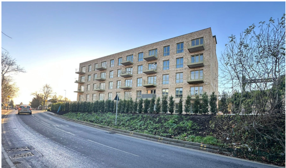
Photo of development as-built from Station Road
