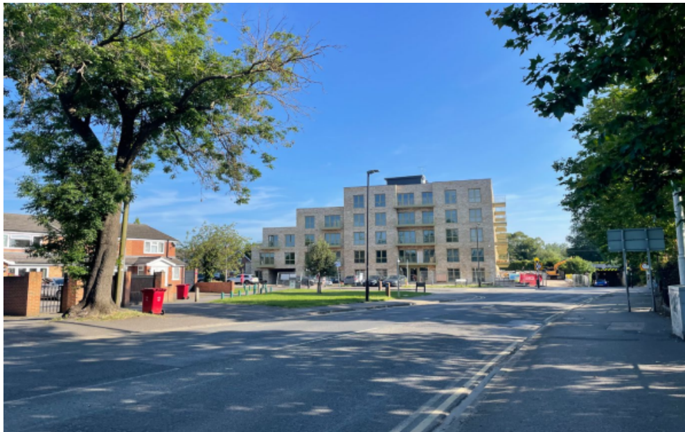
Photo of development as-built looking north along Station Road
