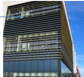
Brise soleil and office glazing
