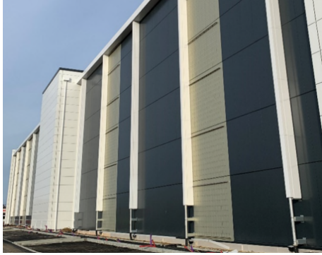
Photo of Building A under construction
