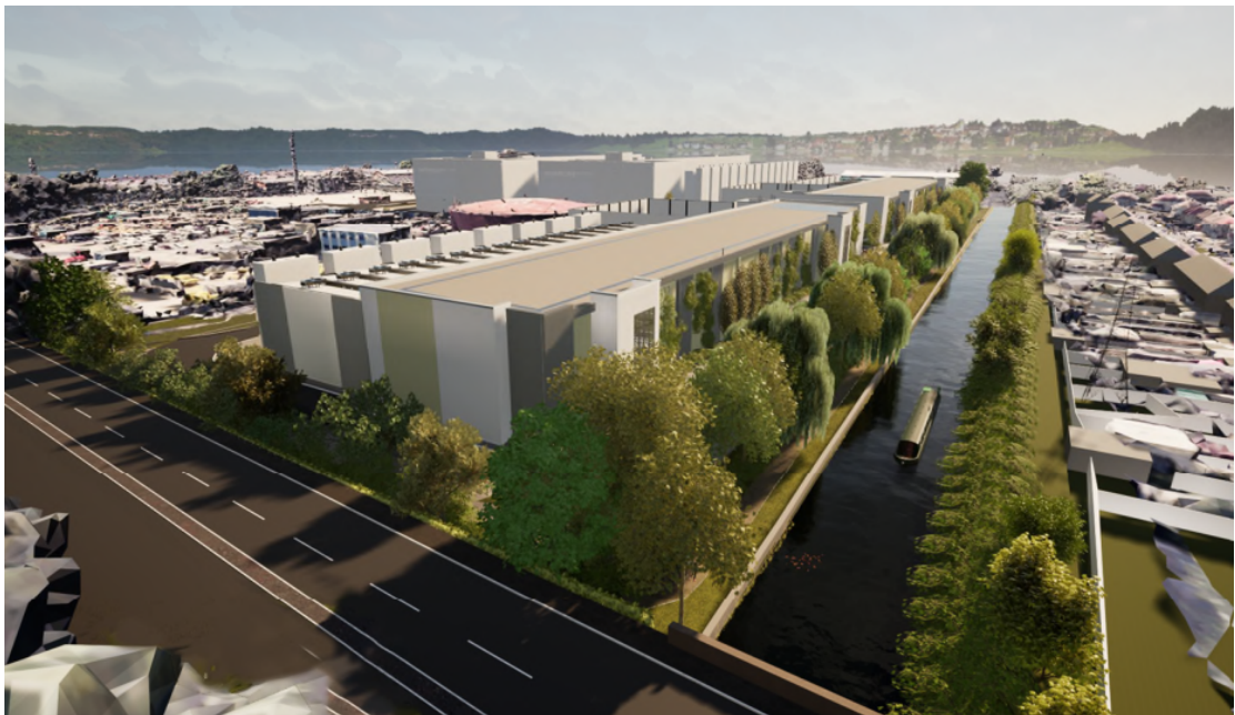
View of Building C and canal looking west with Buildings A and B in background
