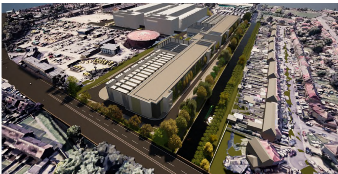
Aerial view of Building C in foreground and Buildings A and B in background
