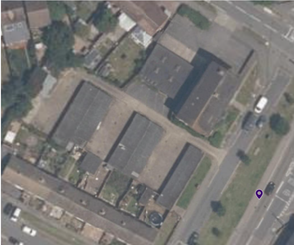
Above image: Slough GIS Aerial Image 2019.
