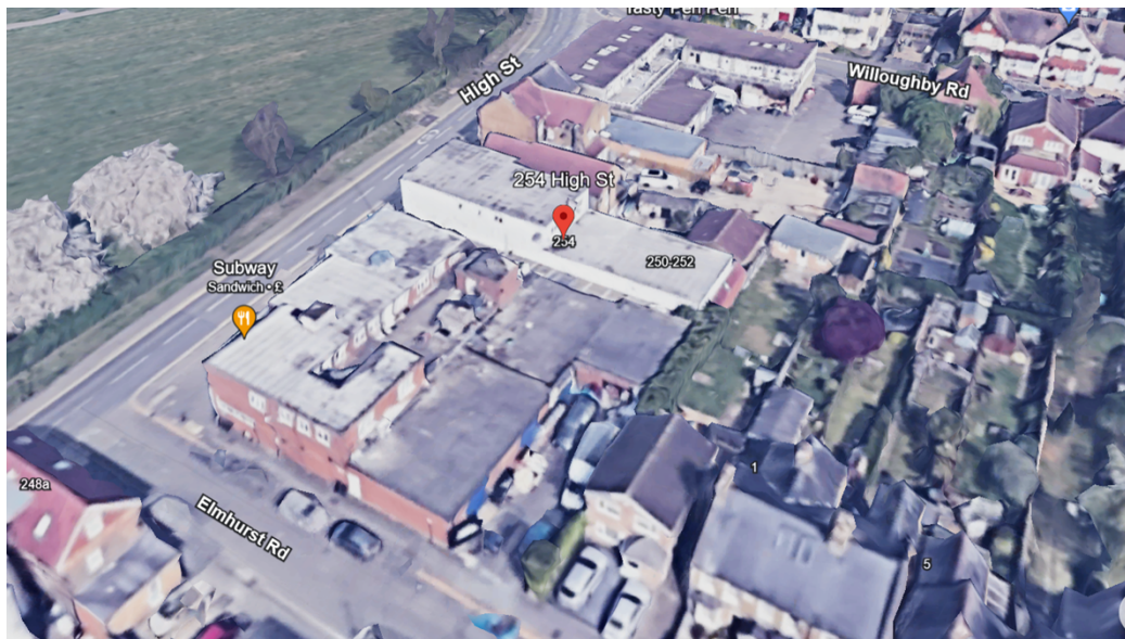
Aerial view looking north across site and neighbouring land/property
