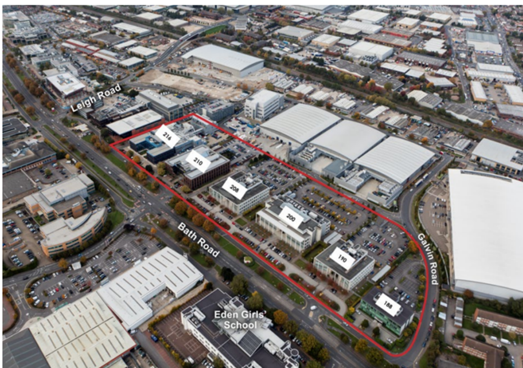
Aerial photograph of site and existing buildings looking north-east
