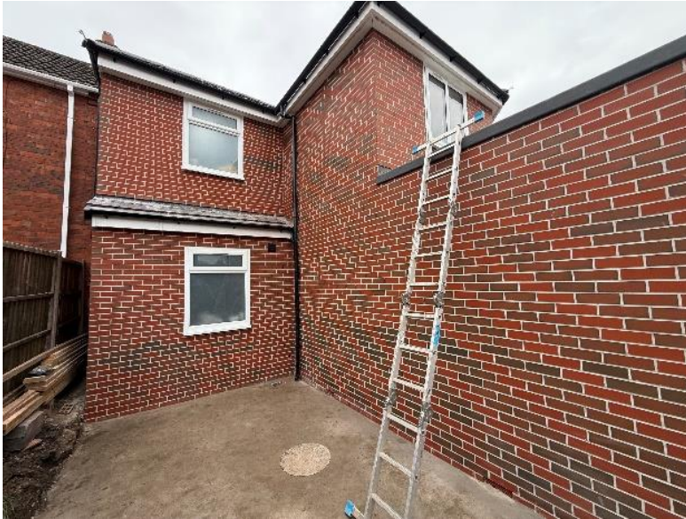
Fig 3 Brick slips applied
