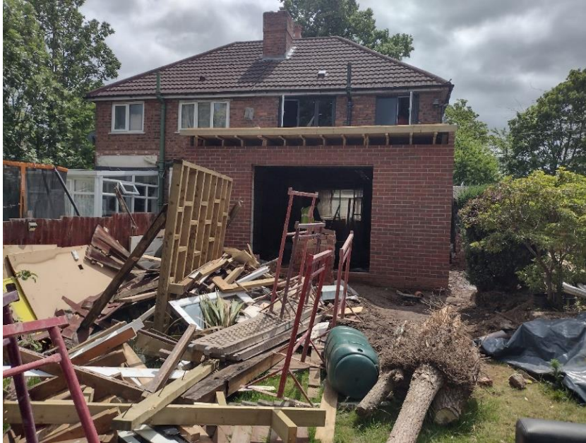
Fig 1 - Rear elevation showing PD/24/02804 (Proposed single storey rear extension measuring: 4.32m L x 2.92m H (2.92m to eaves)).
