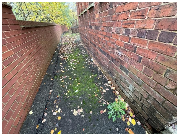
Photo 4 - Cracking to Tarmac suggests Footing Issues to Wall
