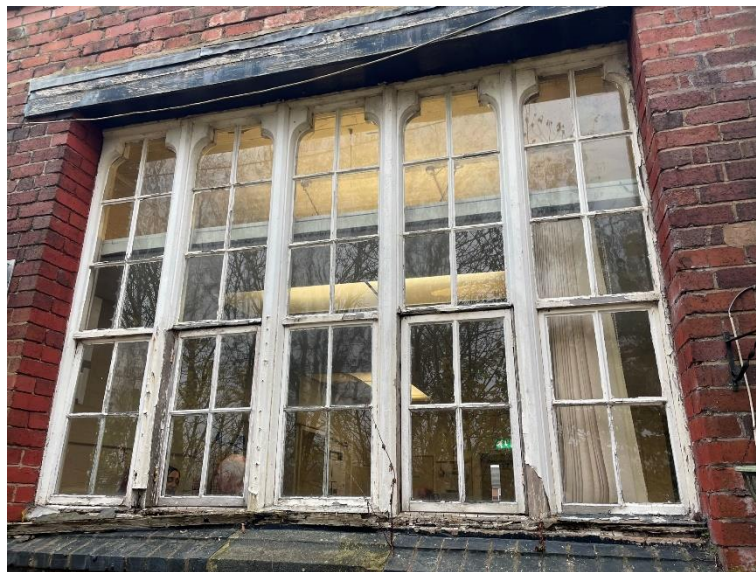
Photo 2 - Poor Condition Timber Window
