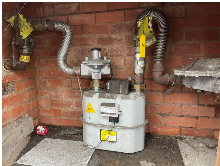
Photo 8 - Gas Meter with Corroded Pipework
