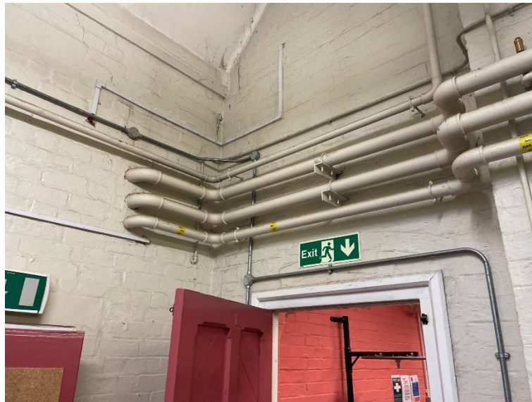
Photo 11- Uninsulated Pipework
