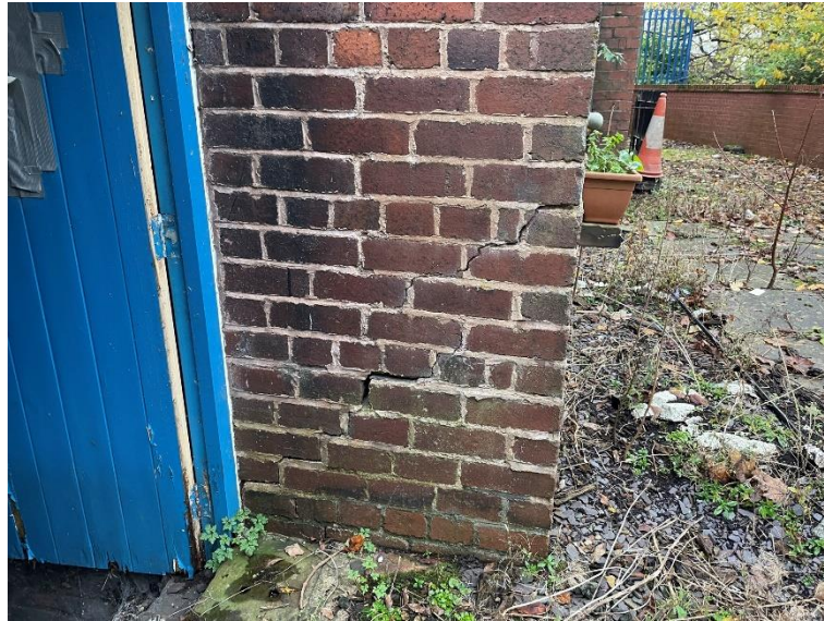
Photo 3 - Stepped Cracking
