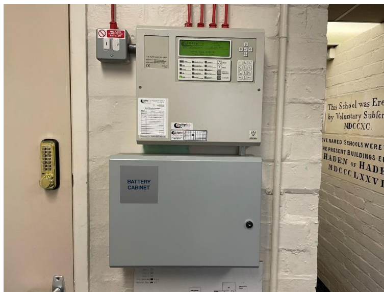
Photo 9 - Fire Alarm Board
