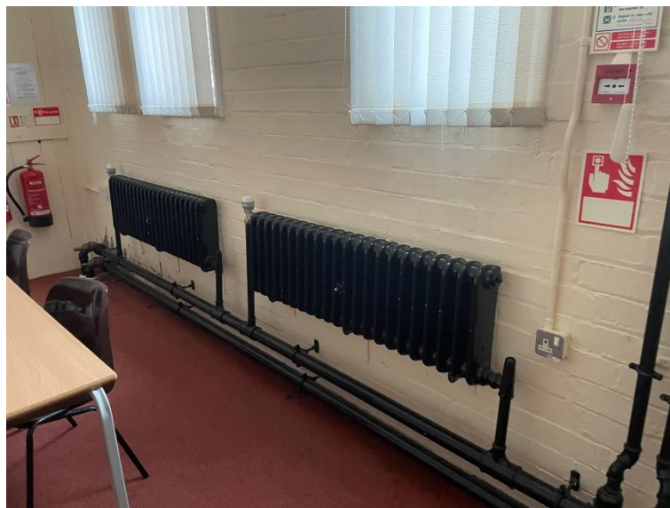
Photo 14 - Exposed Cast Iron Radiators
