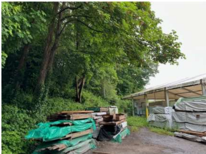
Site photos – DC/24/69156
