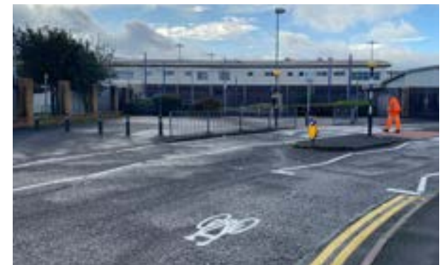
Figure 17 Key Public Realm Areas and Features 1. Market Place 2. Union Street 3. Public realm at Wednesbury Great Western Street metro stop
