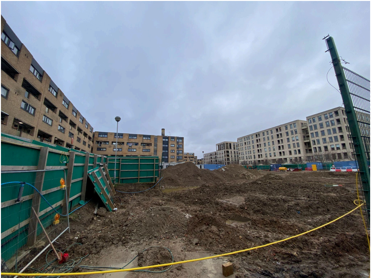
Site of DZ4, open space and DZ5, looking west:
