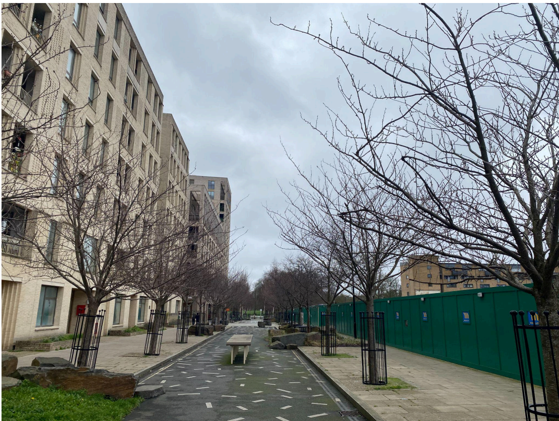
Looking east down Murrain Rd play street (DZ4 site on right, phases 1 and 2 on left):
