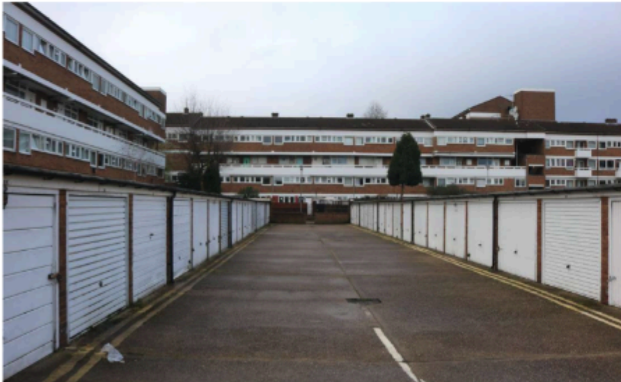
3: The garages seen from the eastern end of the site.
