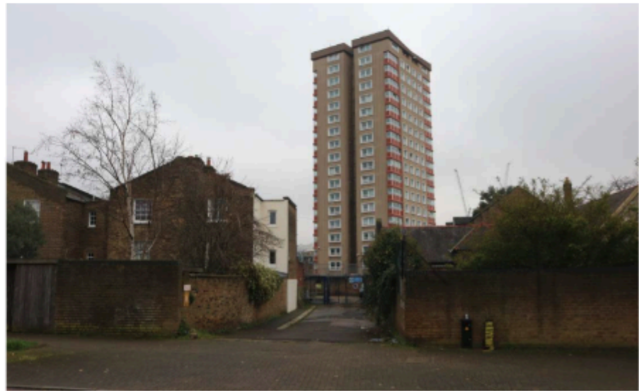
4: Entrance to Welshpool Depot from Tredarwen Road
