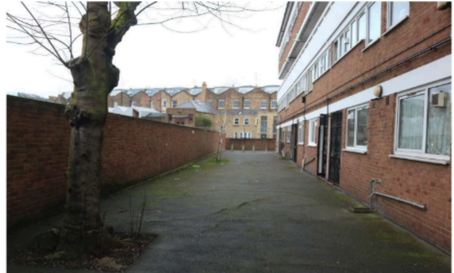
4: Looking east from the entrance of 91 - 104 Orwell Court ("Little Orwell").
