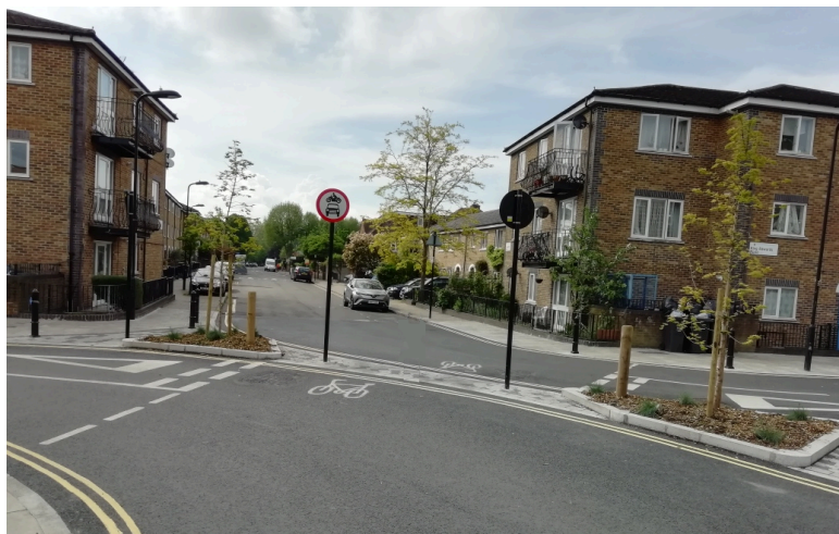
Fig 5.2 Example of a diagonal traffic restriction.
