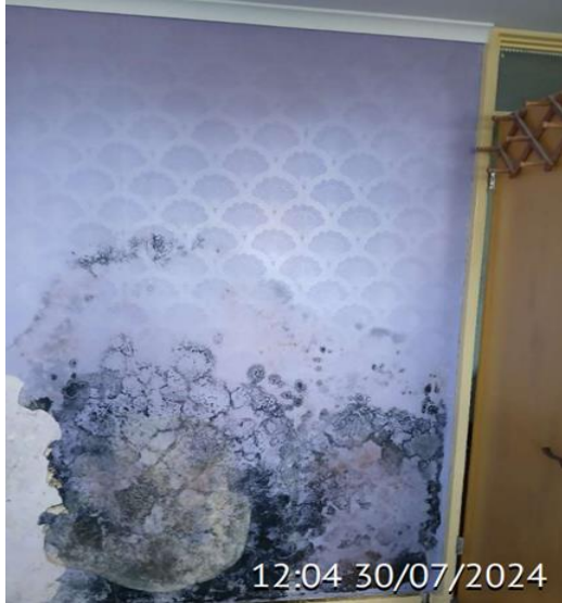
Dering Road- before photos
