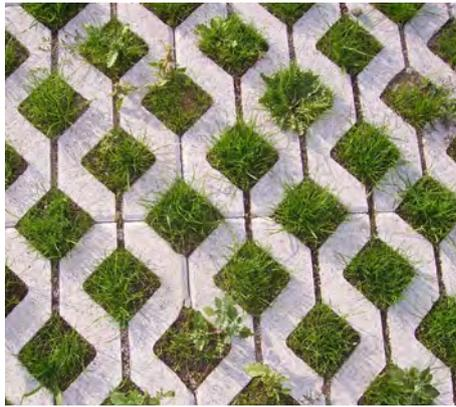
Figure 2.36e: Permeable paving.
