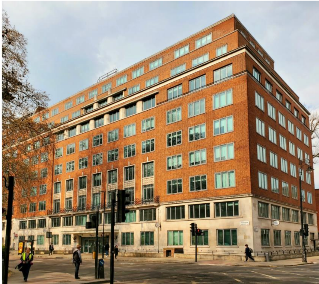
Figure 2: Street view of front elevation
