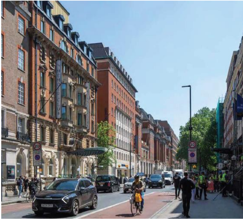
Image 2 – Development from the north on Upper Woburn Place
