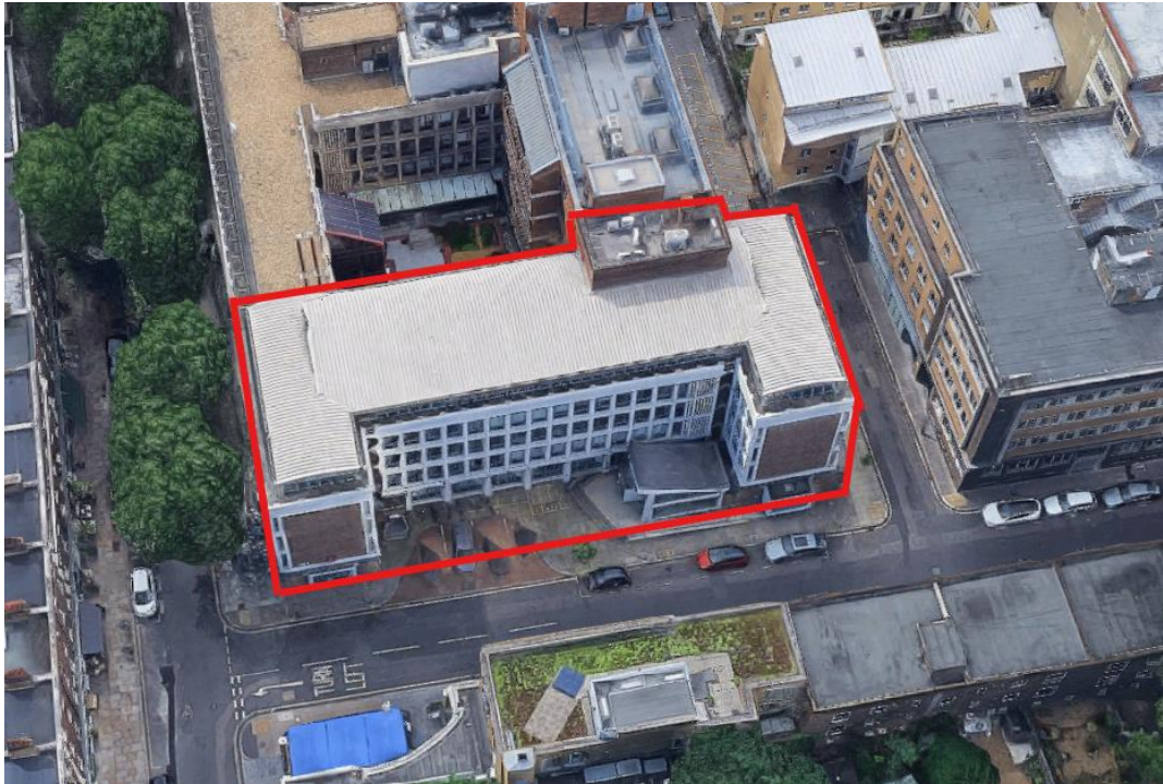
Figure 1 – The existing site with Ridgmount Street in the foreground
