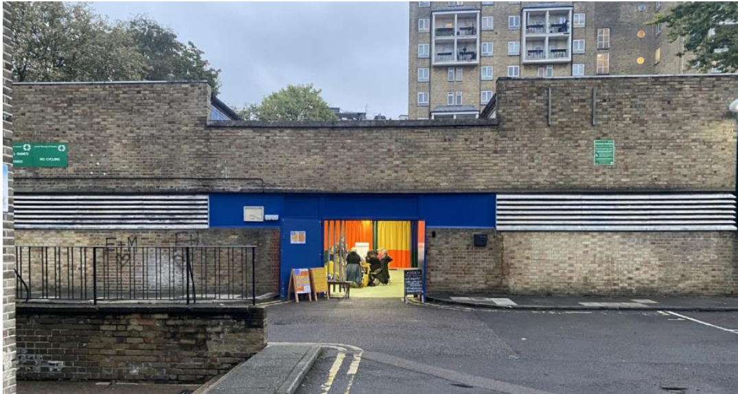
Figure 1 – The existing site
