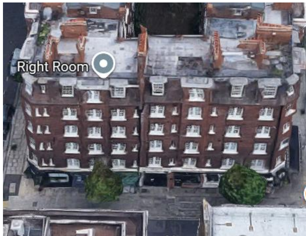
Sinclair House (Residential flats)
