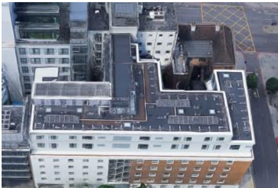
Figure 12 – aerial photo of 79-81 Euston Road
