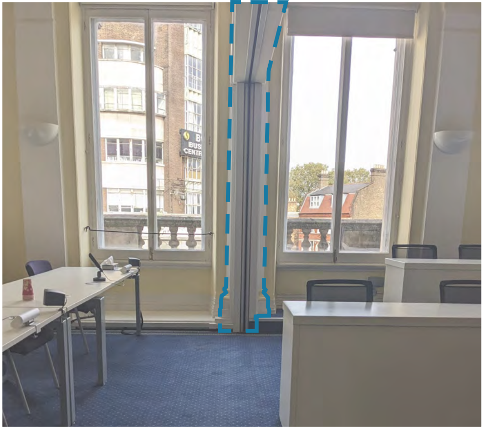
Top: Bulkhead diving the Courtroom on the First Floor Bottom: Sliding partition and bulkhead diving the Courtroom on the First Floor
