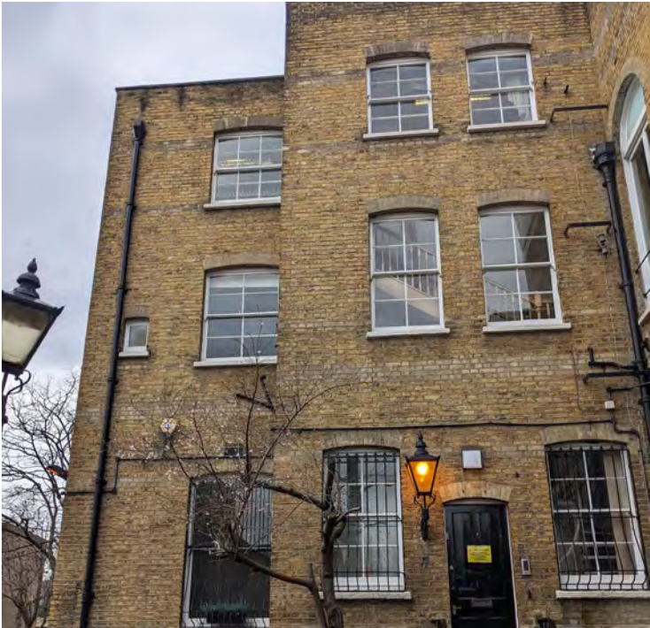
Existing Rear Windows on Bromley Public Hall
