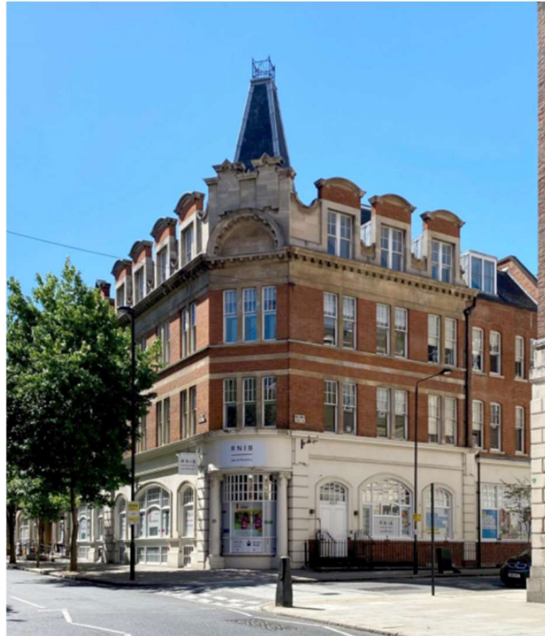
Figure 1 – Street view south on Judd Street of the existing building
