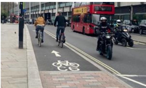
Figure 3.6: Physically separated cycle lanes (this can be done using stepped tracks-wands – as shown in the image- ,kerbs or wands-stepped tracks-and kerbs)
