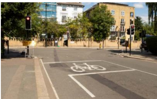
Figure 3.10: Advanced stop line for cyclists
