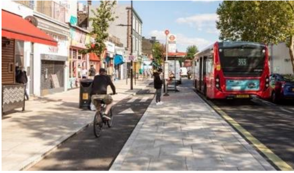
Figure 3.7: Cycle bypass for cyclists at a bus stop
