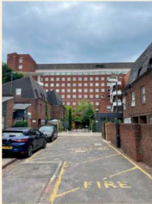
North Facade - Brookes Court
