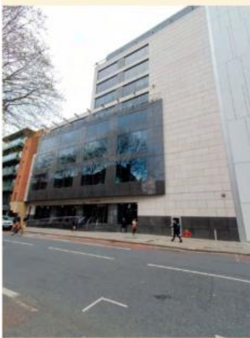
West Facade - Gray's Inn Road
