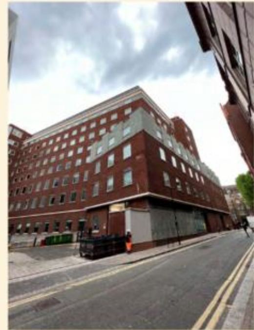
South & East Facade - Brooke Street
