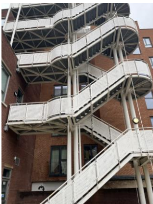
Figure 20: Rear of 24-28 Gray's Inn Road
