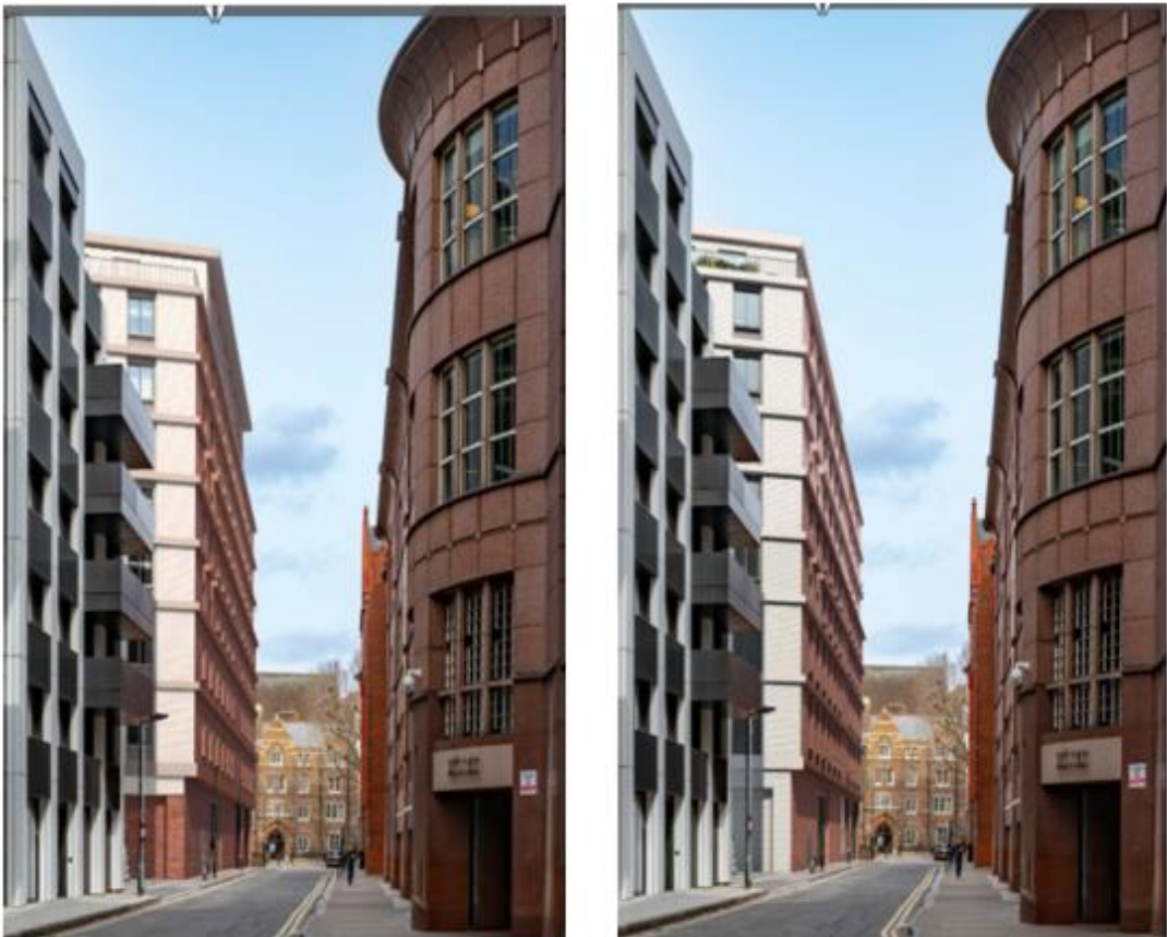
Figure 12 (Left) Original view from Brooke Street (Right) Amended view from Brooke Street
