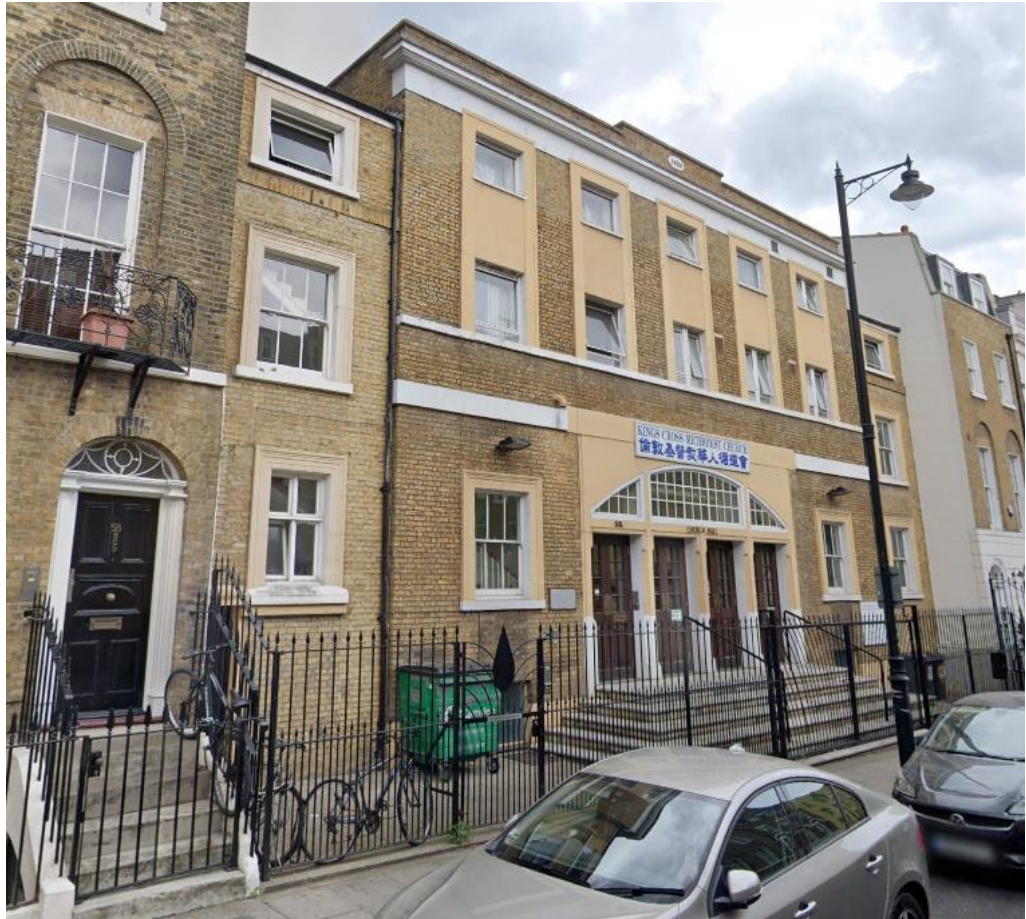
Figure 1 – The existing site as viewed from Birkenhead Street
