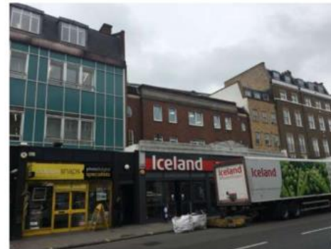
View of 301-305 Kentish Town Road
