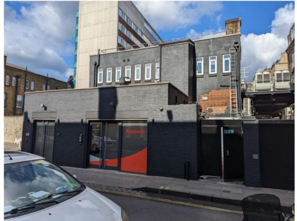
View of existing office entrance on Holmes Road
