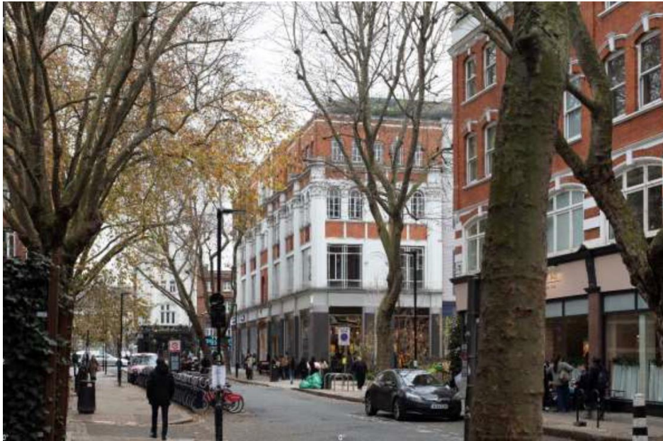
Figure 11 – Image of the roof extension from Store Street in winter months
