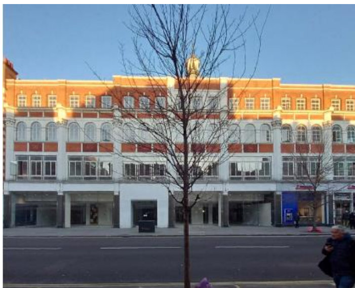
Figure 7 – View of site from Tottenham Court Road
