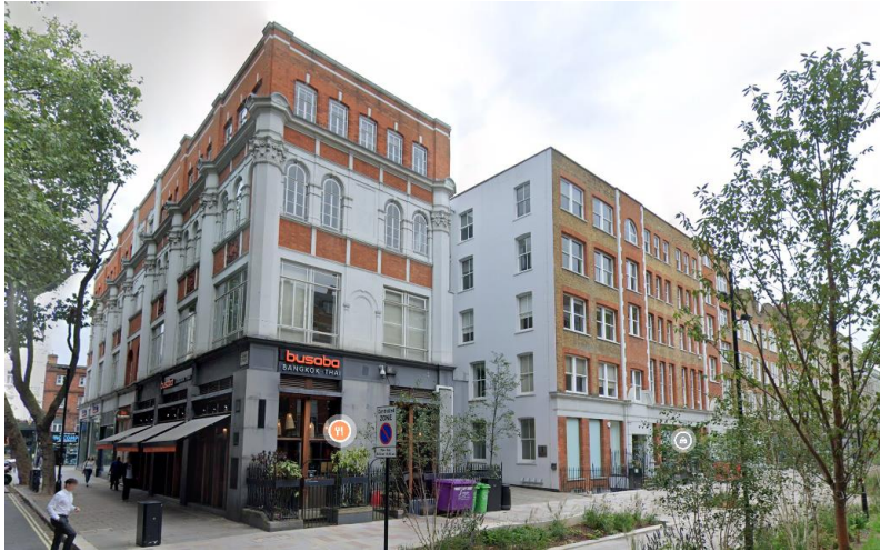
Figure 5 – View of site from corner of Alfred Place and Store Street
