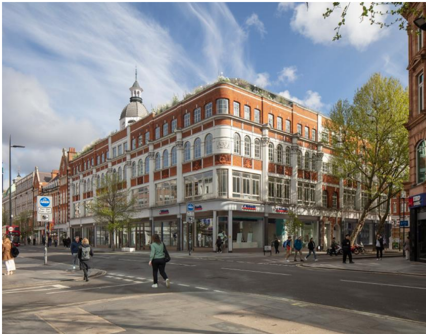
Figures 12A (top) & 12B (bottom) – Images of the existing and proposed site with roof extension and relocated cupola visible
