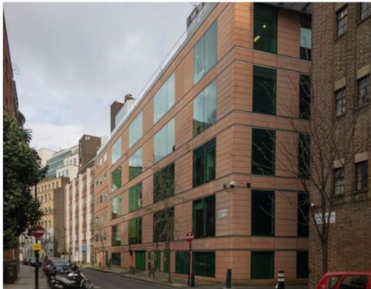
Figure 5.2: The existing building upon the site from New Compton Street
