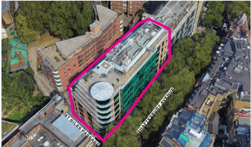
Figure 1 – The existing site
