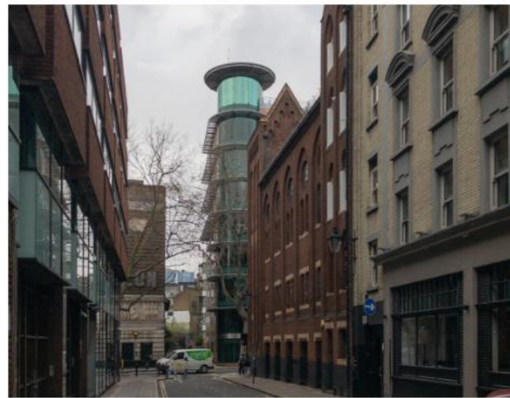
Figure 5.3: The existing building upon the site from Mercer Street
