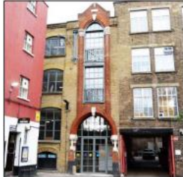
5. WAREHOUSE WITH OPEN PLAN OFFICES (GRADE II LISTED)
