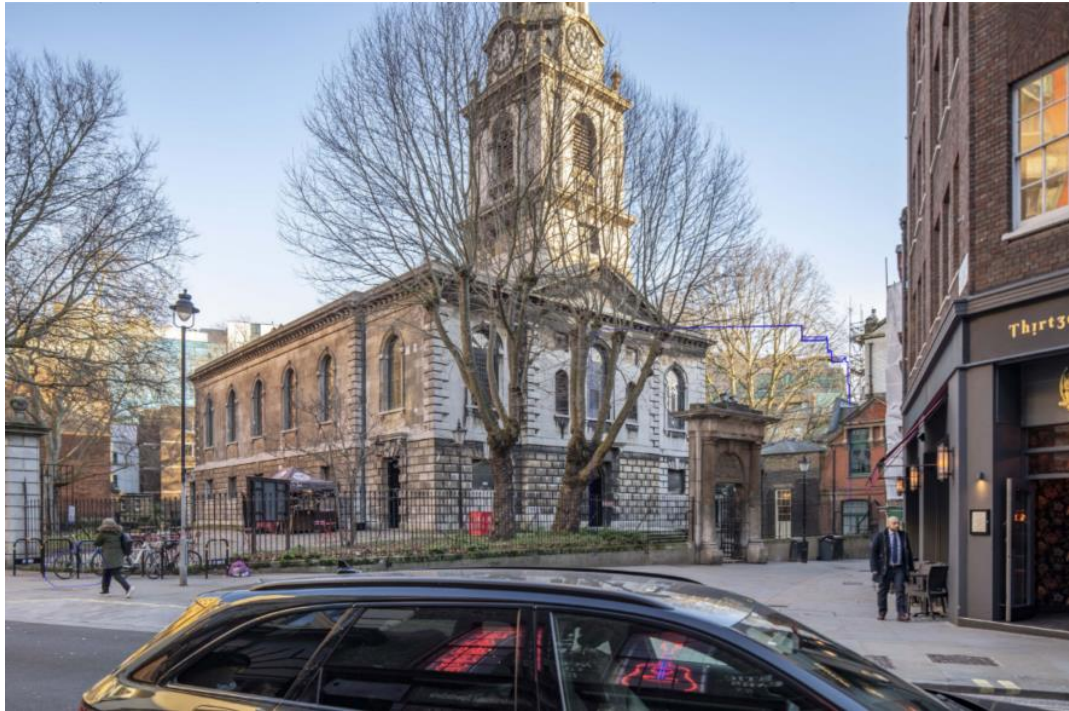
Figure 5: Proposed wireline view of The Church of St Giles in the Fields from Denmark Street
