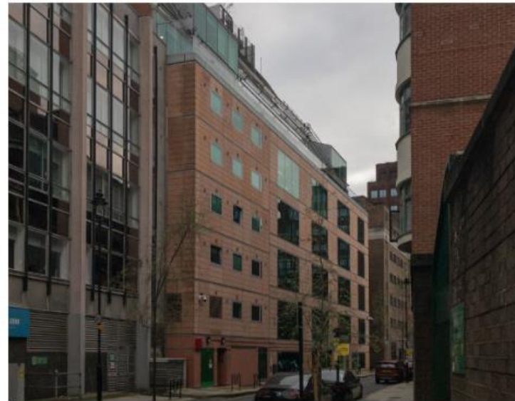
Figure 5.4: The existing building upon the site from New Compton Street
