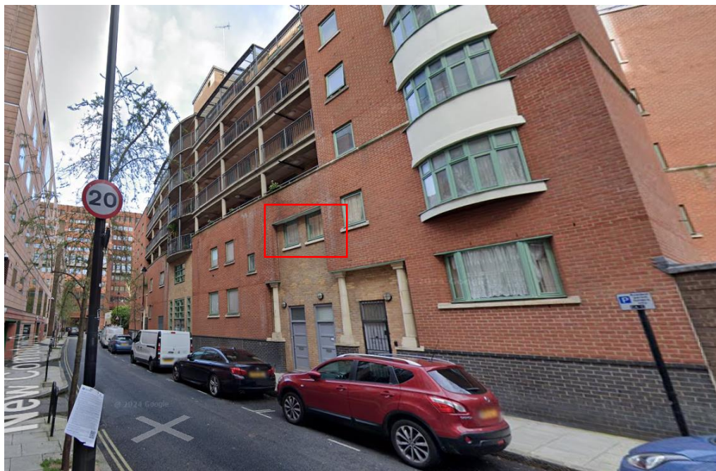
Figure 14: Impacted windows at Pendrell House
